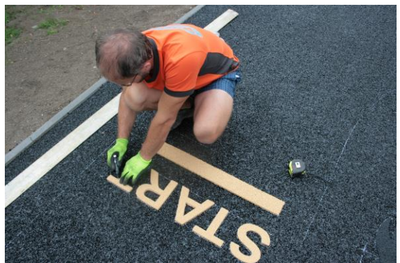
Measure out and copy graphic on cured SBR layer along with requested design.
