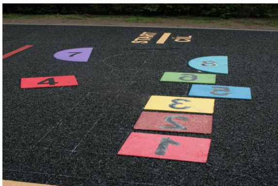
Measure out and copy graphic on cured SBR layer along with requested design.
