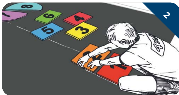
Measure and copy the graphic on a cured SBR layer along with the required design.
