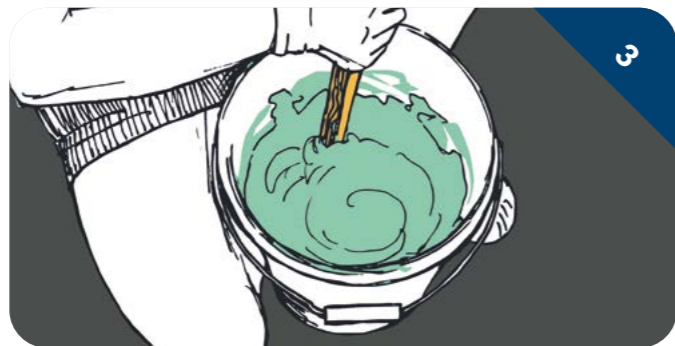
Mix the two-component glue properly. Use standard PU glue for artificial grass. Use the two-component glue for larger patterns or more graphics.
